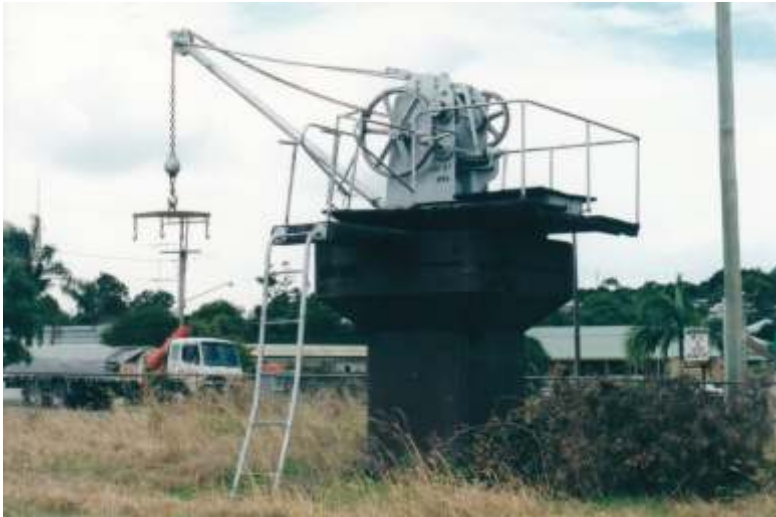
Yard Crane at Cooroy with case lifting adaptor attached.
